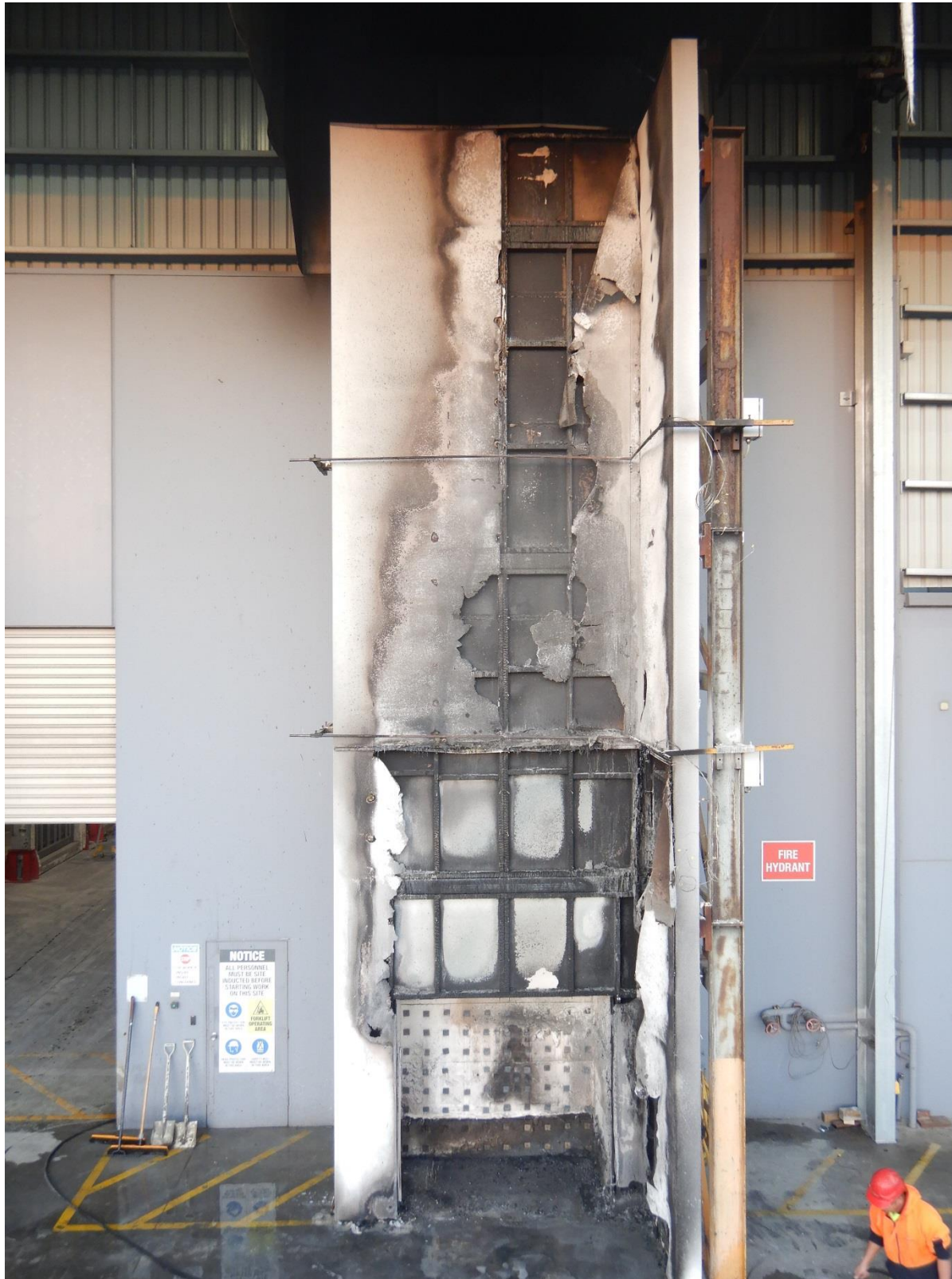
Figure 41 The external wall system on completion of the test – main wall
