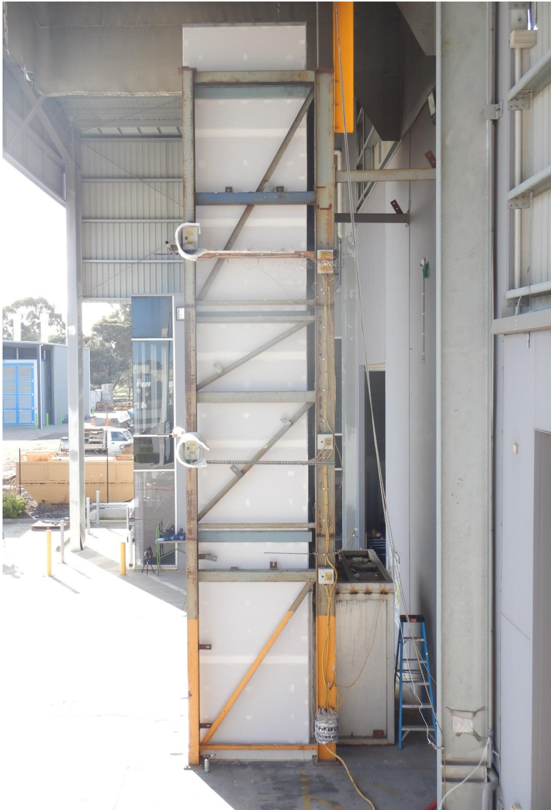
Figure 31 The unexposed side of the external wall system before the start of the test – wing wall
