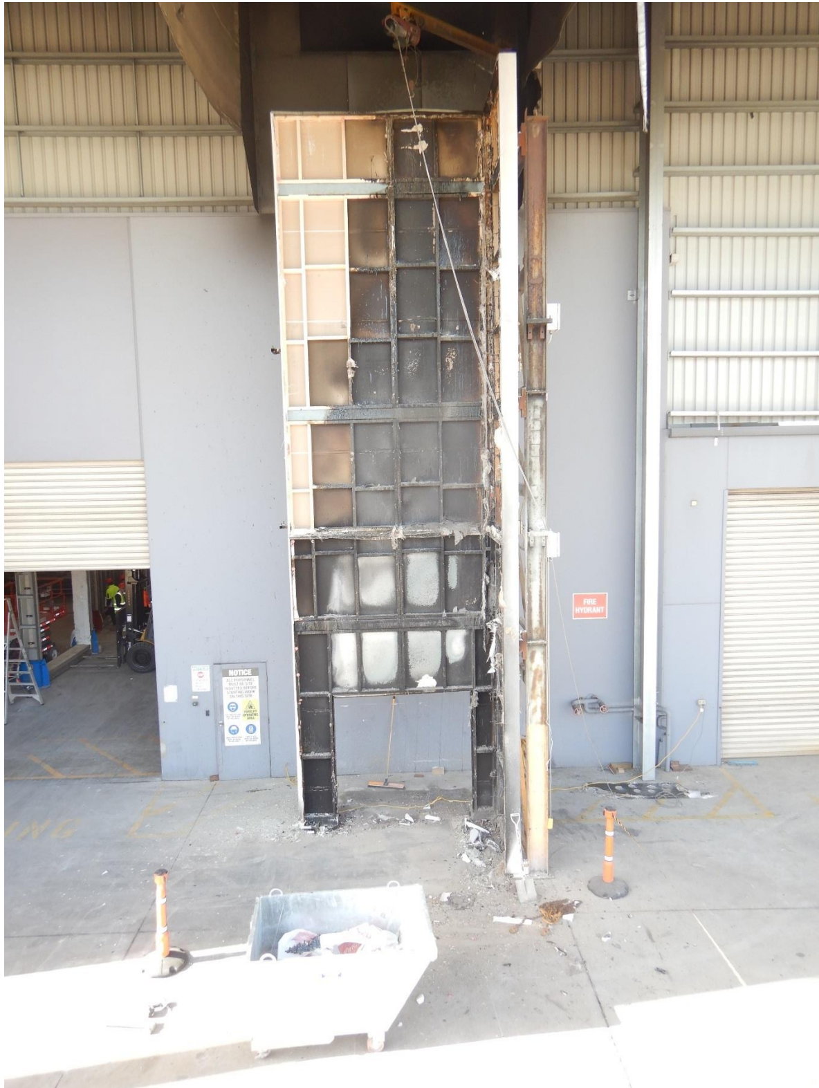
Figure 51 The post-test external wall system with the sarking removed – main wall
