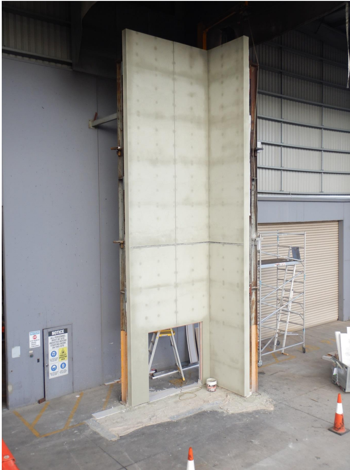
Figure 27 The wall system with rendered (1 st render coat) EPS panels during construction.
