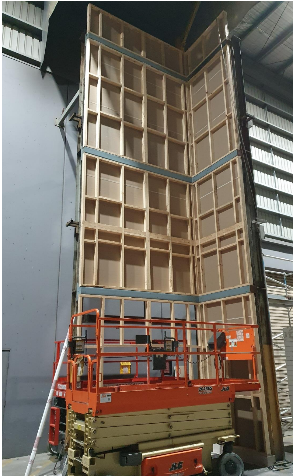
Figure 25 The time framing with plasterboard cladding.
