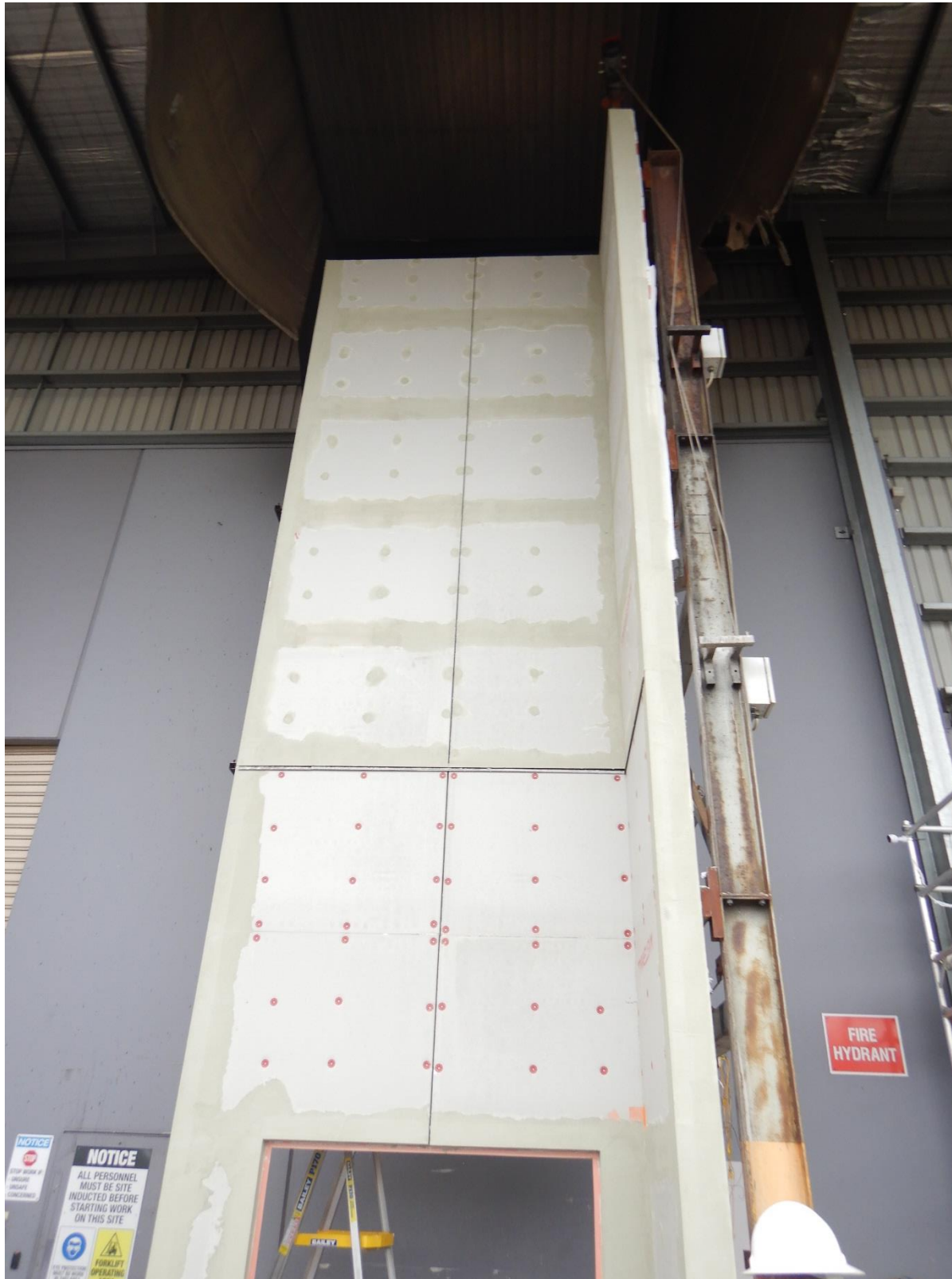
Figure 26 The wall system with EPS panels during rendering.
