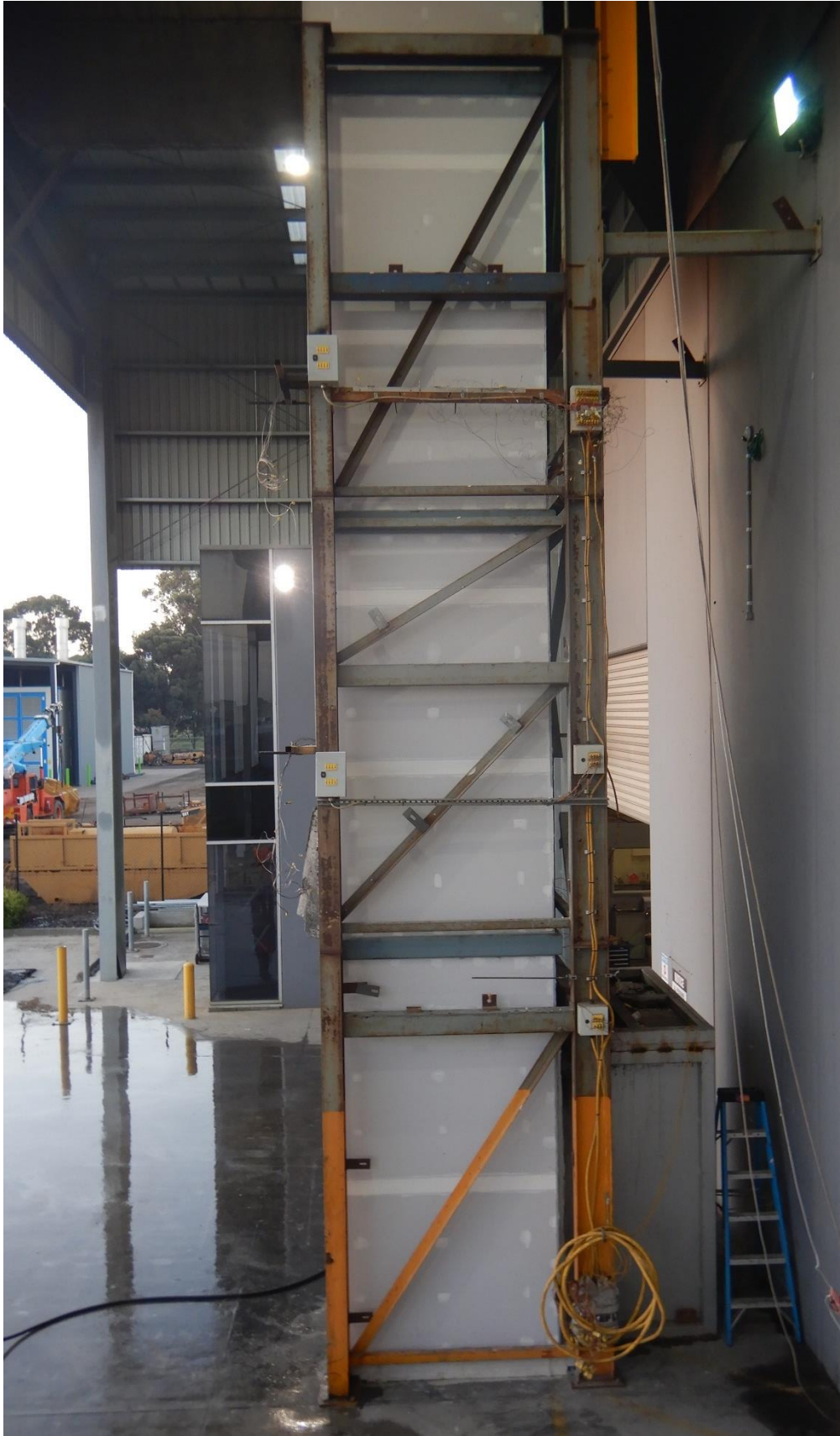
Figure 44 The unexposed side of the external wall system on completion of the test – wing wall
