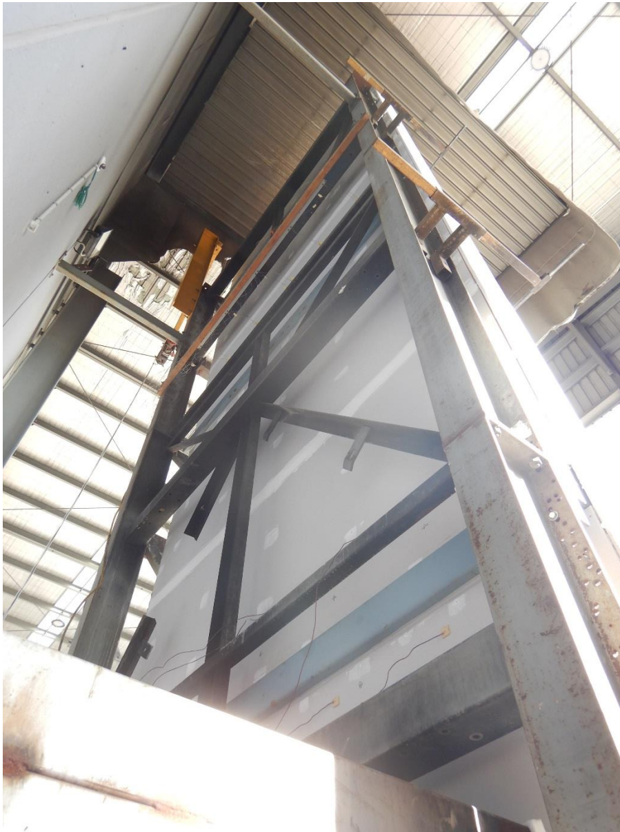
Figure 30 The unexposed side of the external wall system before the start of the test – main wall
