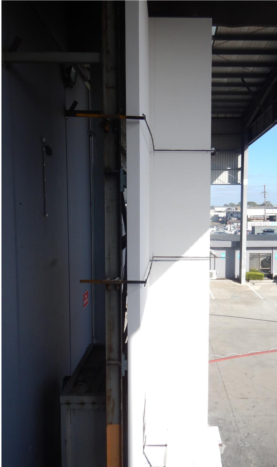
Figure 29 The complete external cladding system before the start of the test – wing wall
