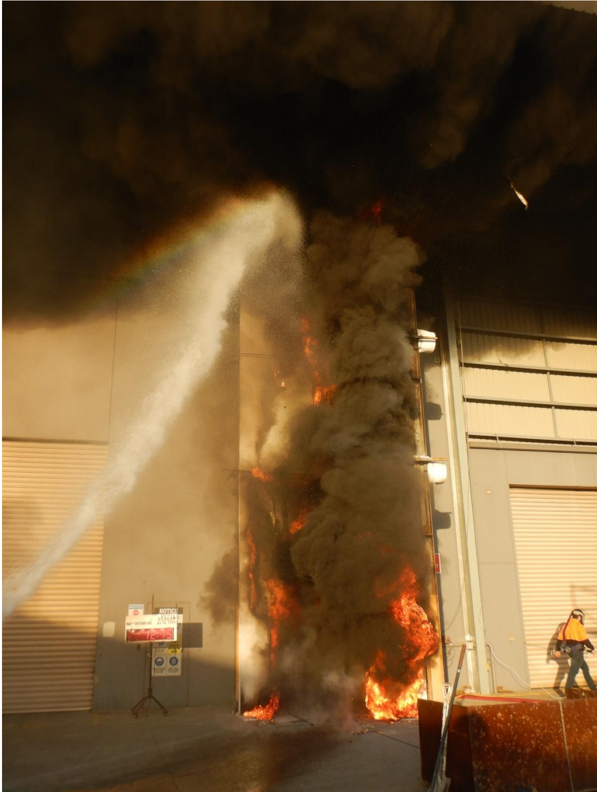
Figure 40 The external wall system at the end of the test.
