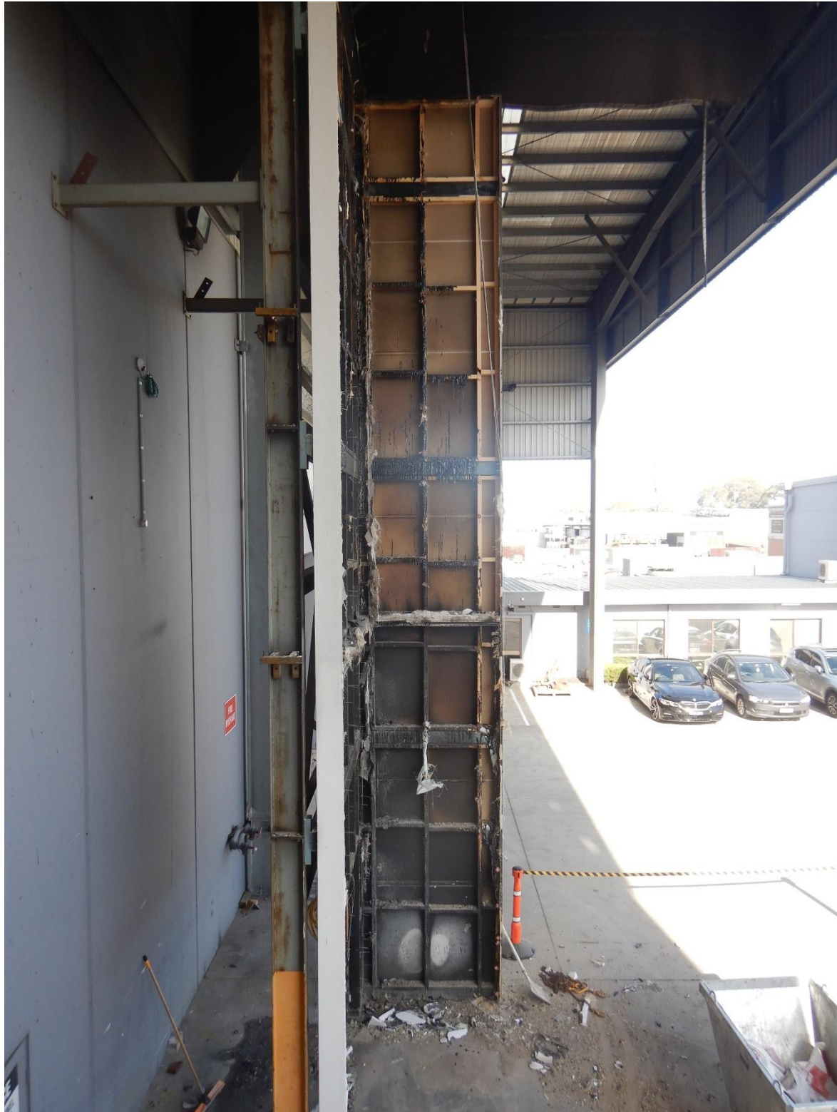
Figure 52 The post-test external wall system with the sarking removed – wing wall
