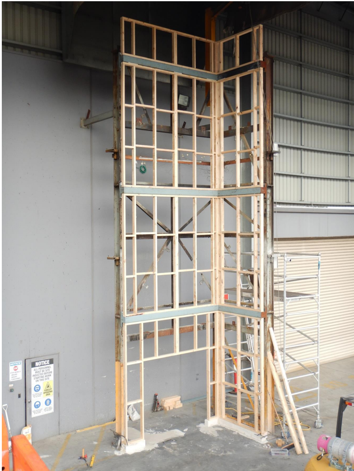
Figure 24 The timber framing during construction – back blocking not present at this stage.
