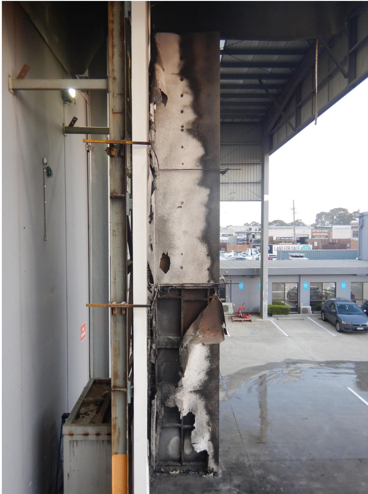
Figure 42 The external wall system on completion of the test – wing wall
