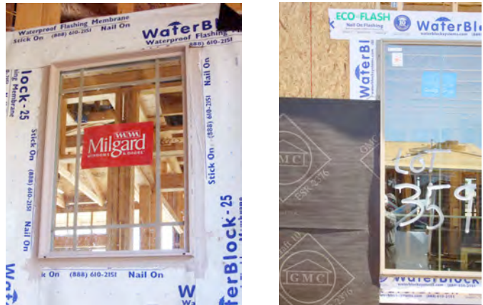
Photograph 1: Gravity Lap Part I (left)– The flashing strips are layered shingle fashion. Horizontal bottom sill first. Vertical side jambs next. Horizontal head flashing last. Note the sealant used to provide water control layer continuity between the window unit and the flashing strips. Photograph 2: Gravity Lap Part II (right)– The rolls of building paper are installed horizontally shingle fashion. The vertical edge of the building paper is sealed to the edge of the window unit with more sealant. Any water that enters at that joint is expected to be controlled by running down the vertical “side flashing” or jamb flashing and out at the bottom. The width of the jamb flashing is problematic. That is why the flashing tape and housewrap detail at the window jamb flange shown in Figure 2 (and in Sidebar I) is such an improvement.
