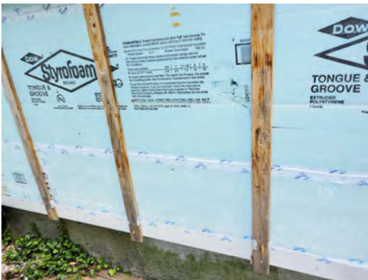
Photograph 8: Wood Sheathing (above left) - Residentially we now use tapes on wood sheathings that have factory applied membranes factory bonded to them to provide water management and air management. Photograph 9: Foam Sheathing (above right) - Foam plastic sheathing panels are taped together creating a water-resistive barrier system. These systems are now around 20 years old. This image dates back to a subdivision development in Chicago in 1995. 3M was one of the first to develop acrylic based tape system for housewraps in the 1980's and they migrated to foam sheathings in the 1990's.
