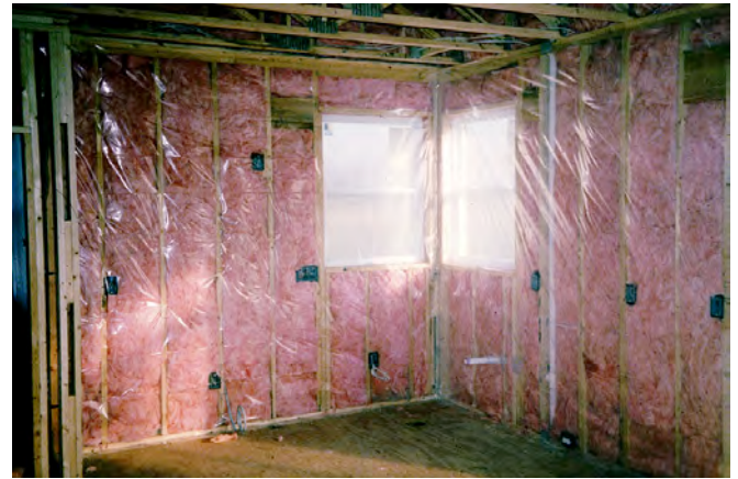
Photograph 3: Interior Polyethylene Vapor Barrier —The sheet polyethylene on the interior is clearly a vapor barrier. In this assembly it is also acting as an air barrier (air control layer).
