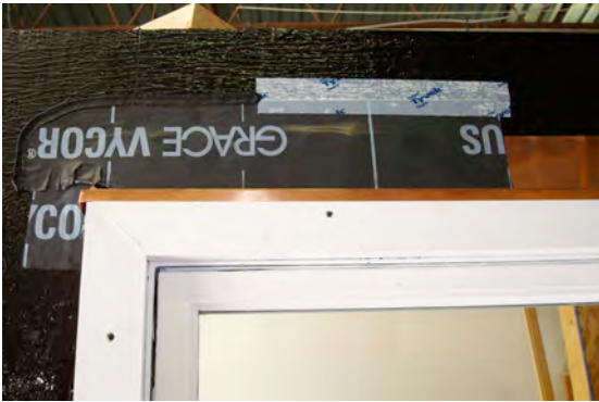
Photograph 14: More Termination (above left) - With flashing tapes we tend to terminate them two ways – with either a sheathing tape or a bead of sealant. A sheathing tape does not need to be terminated – it terminates itself. Figure 4: Termination of Flashing Tape (above right) – The “red” horizontal tape is a butyl based “flashing tape” that is “terminated” by a “green” acrylic based “sheathing tape.”
