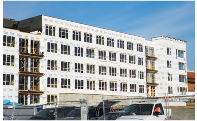
Photograph 3: Multifamily —Sheet vapor permeable water control layer and air control layer. The “classic” air infiltration barrier that also controls rainwater installed on the exterior of vapor permeable sheathing such as glass faced gypsum board.
