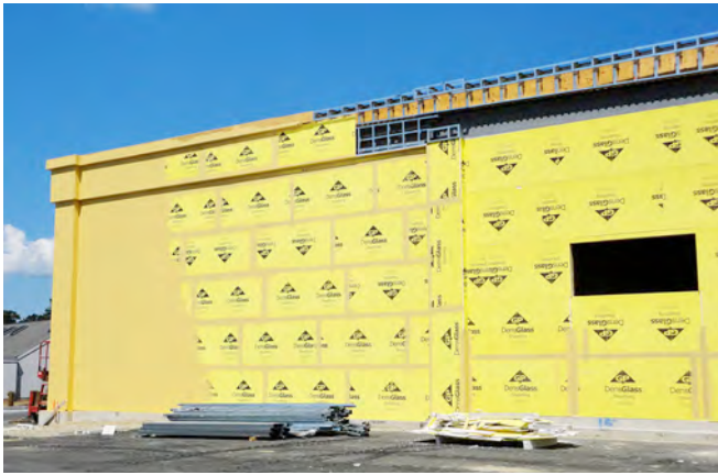
Photograph 2: Commercial/Retail —Fluid applied vapor permeable water control layer and air control layer installed over a vapor permeable glass faced gypsum board.
