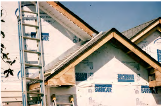
Photograph 14: More Termination (above left) - With flashing tapes we tend to terminate them two ways – with either a sheathing tape or a bead of sealant. A sheathing tape does not need to be terminated – it terminates itself. Figure 4: Termination of Flashing Tape (above right) – The “red” horizontal tape is a butyl based “flashing tape” that is “terminated” by a “green” acrylic based “sheathing tape.”
