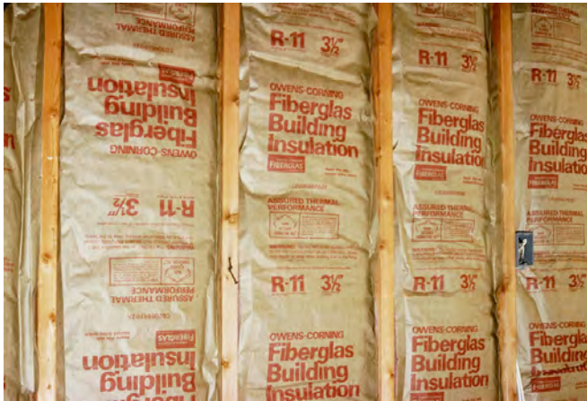
Photograph 4: Kraft Faced Fiberglass Batts —The facing is the vapor control layer. Note that the Kraft facing does not function as an air barrier (air control layer).
