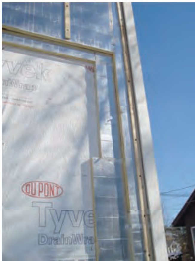
Photograph 7: Vapor Closed Foil Faced Continuous Exterior Insulation – Note the draining building wrap providing redistribution of moisture. And, yes, we were also here earlier...”Joni Mitchell, Water and Walls, ASHRAE Journal, August, 2013).
