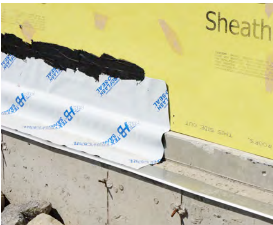
Photograph 7: Termination (left)– This “terminate” the reverse lap thing is a big deal. A continuous bead of sealant is used to glue the top edge of the reverse lap to the underlying membrane or sheathing.
