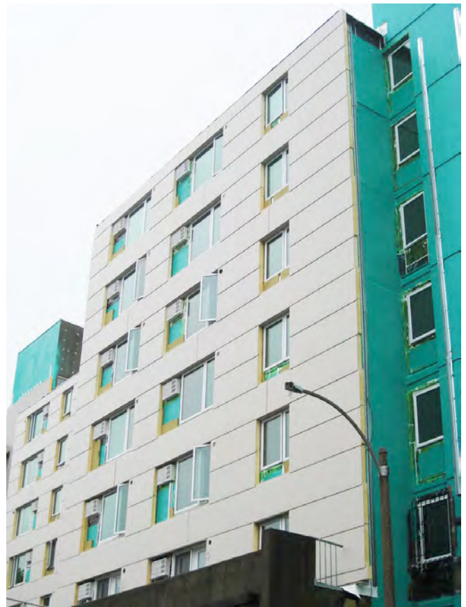
Photograph 7: Retrofit Metal Panel —Insulated metal panels only provide the thermal control function and cladding function.
