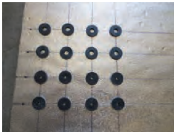
Photograph 8: Cap Nails/Washers - Gaps of 1/32 to 1/16 of an inch have a huge positive benefit. Note that the spacing needed to be small to limit the reduction in thermal performance of the exterior continuous insulation.
