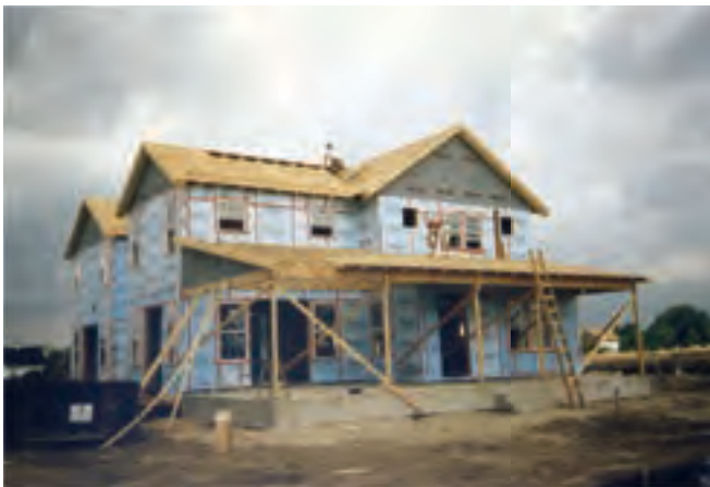
Photograph 4: Vapor Closed Exterior Continuous Insulation - If you used a vapor closed exterior continuous insulation like extruded polystyrene drying to the exterior was not possible.
