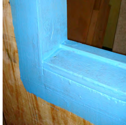
Photograph 3: Formable Flashing (above left) – Life got better when flashing systems became formable and flexible. This photo dates back a decade to when I got my first sample of flexible flashing to play with in my back yard. I thought it was the greatest invention since the transistor. Ok, so I am exaggerating - but only a little. Look at how beautifully a seamless under window flashing system is created. Photograph 4: No Origami Here (above right) – Today's liquid applied systems easily handle complex geometries seamlessly.
