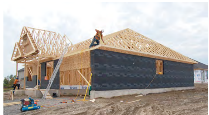
Photograph 1: Residential —Fully adhered vapor permeable water control layer and air control layer. Yes, one material or product can do both things. Note the now typical oriented strand board (OSB) sheathing—a semi-vapor permeable material—an “external vapor throttle”.
