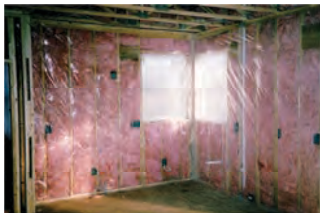
Photograph 2: Polyethylene Vapor Barrier – a "classic" Class I vapor retarder. Also a pretty darn good air control layer when installed with fastidious care...
