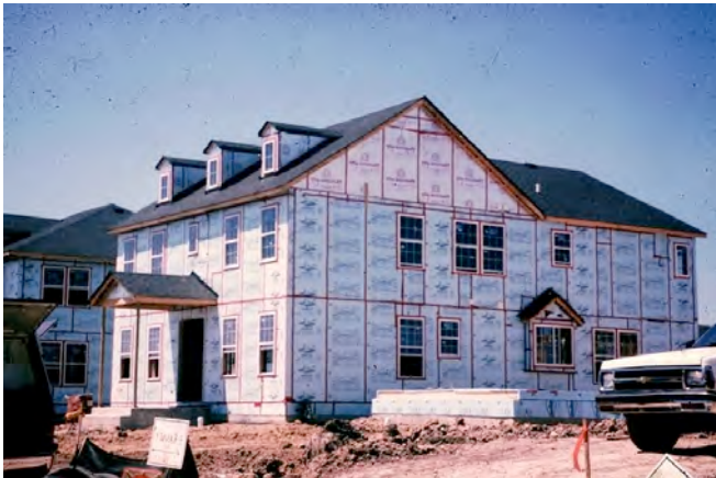
Photograph 2: “Classic” Wood Frame Wall With Foam Sheathing —A wall that we have been building in cold climates for 40 years. The foam sheathing on the exterior is clearly a vapor barrier. The “vapor profile” is that of a “double vapor barrier”. I grew up with this wall in Ontario—2x6 wall with R-5 foam sheathing and a plastic interior air/vapor barrier.
