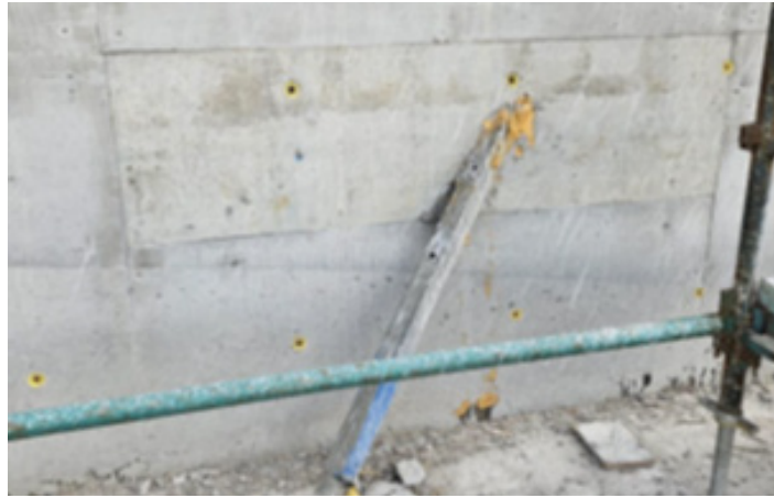
Figure 14: In situ wall with temporary prop cast in.
