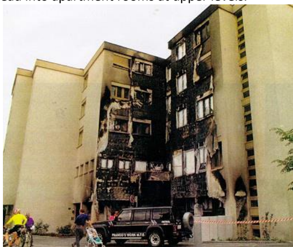
Figure 49 - Munich EIFS fire 1996 [78]
