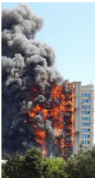
Figure 42 - Baku High Rise residence fire, Baku, Azerbaijan (2015)
