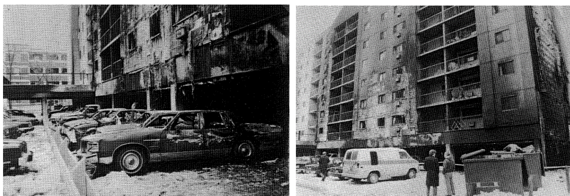
Figure 50 - Damaged cars outside east wall (LHS) and extent of damage to east and north walls (RHS) [82-84]
