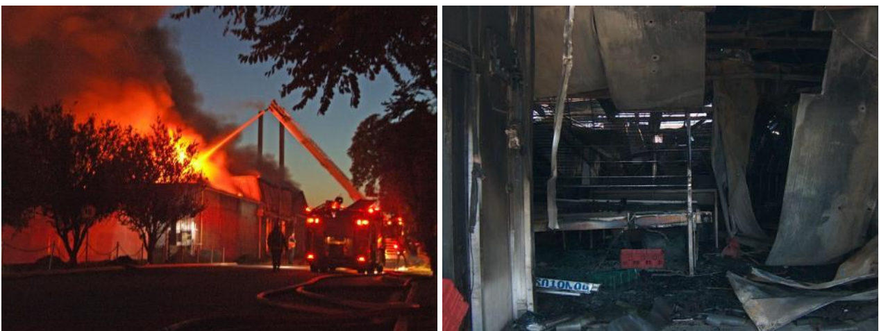
Figure 53. Tegel factory fire 2007 [90]
