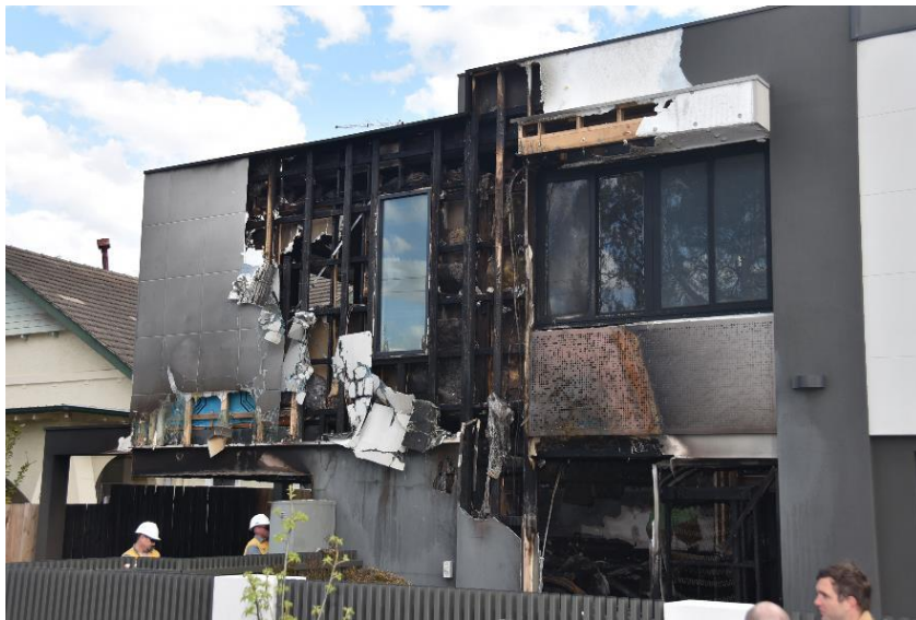
Figure 33 - Post fire damage to street frontage shown on two storey unit (Photos provided by MFB)
