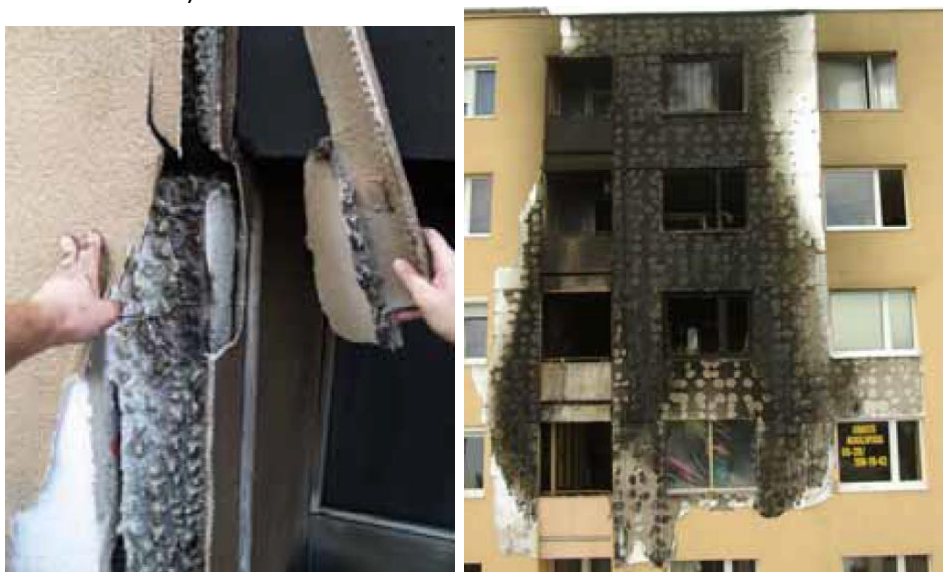
Figure 46 – EIFS fire in Miskolc showing damage to cladding (LHS) and extent of damage to façade (RHS) [81]
