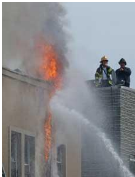
Figure 43 -Flames burn vigorously above the roof line of the EIFS-clad structure (left), View of opposite side of building (away from area of fire spread) [78]
