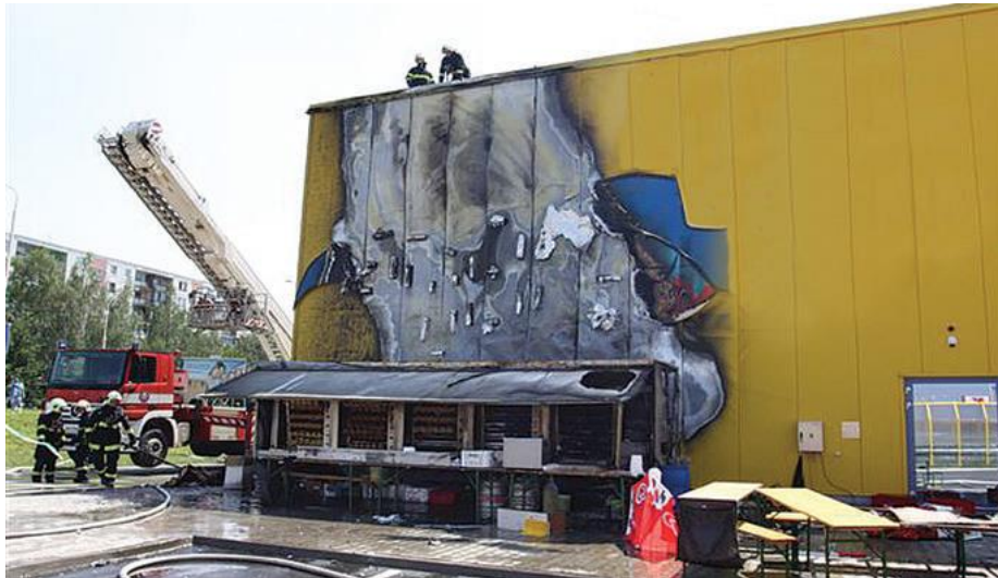
Figure 56 – PIR Insulated Sandwich panel post fire damage on Furniture Retail Warehouse, Slovakia
